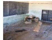
... a class room in need of help...
